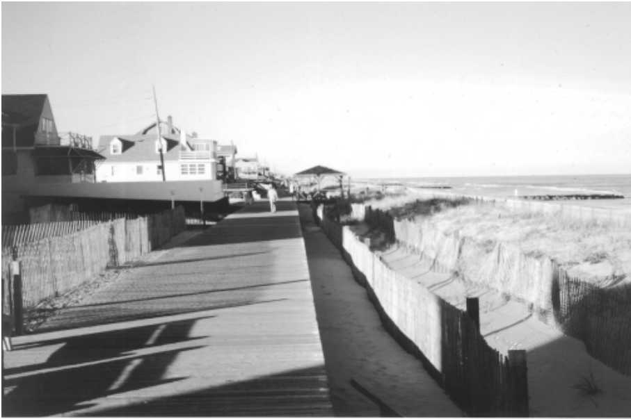
Fig. 3. Linear dune created for shore protection at Lavallette, New Jersey. The fence between the landward side of the dune ridge and the boardwalk was emplaced subsequent to the dune construction project to prevent besanding of the boardwalk.
